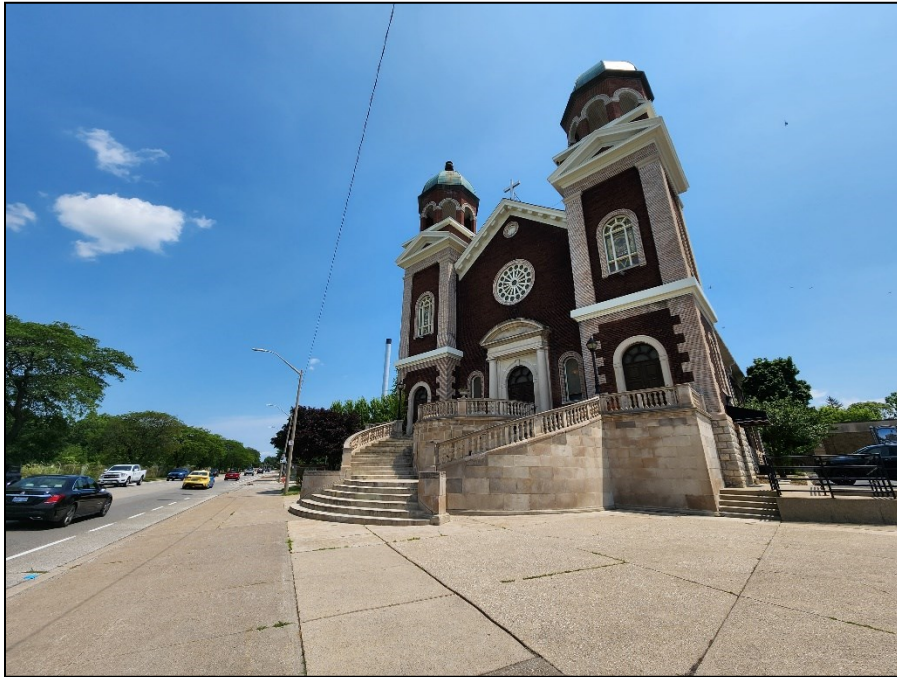
Plate 3: Oblique view of the north elevation, with Riverside Drive East at left, looking southeast (A.S.I. 2023)
