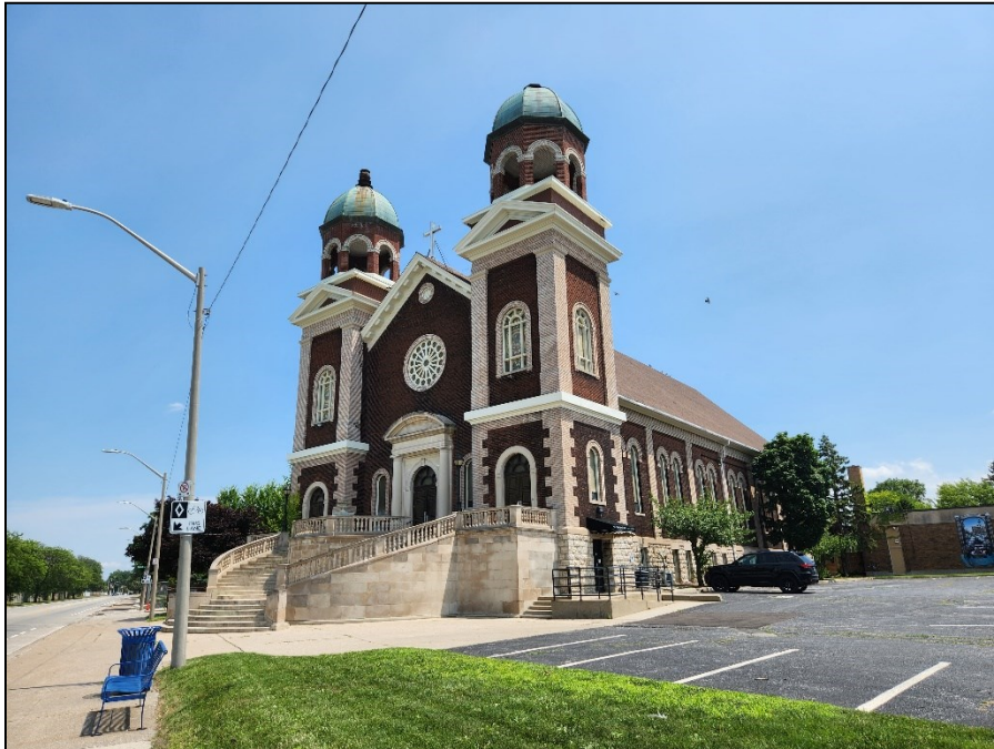
Plate 5: Oblique view of north and west elevations, looking southeast (A.S.I. 2023)
