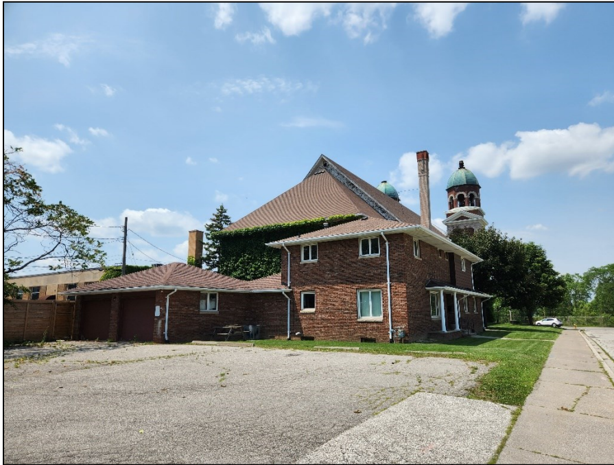
Plate 9: South elevation, with original church structure covered in ivy at left, and later addition at right. Note the parking lot in foreground and garage at rear left (A.S.I. 2023)
