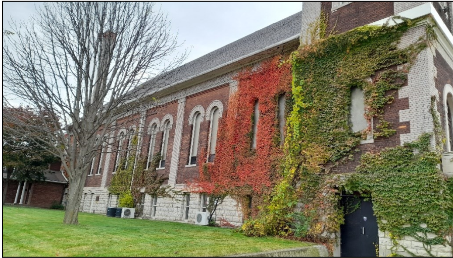
Plate 7: Oblique view of the east elevation, with southern addition at far left, looking southwest (A.S.I. 2023)
