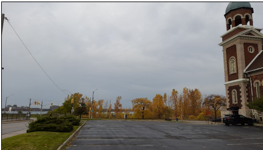
Plate 10: Western parking lot, with the western tower on the northern elevation visible at far right, looking north. Note Drouillard Road to the far left (A.S.I. 2023)
